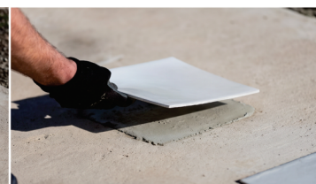
PLACING SECOND PAD
